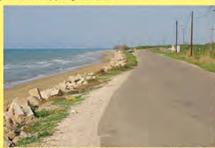
The remnants of the Othoman levee can be distinguished as fresh water can be seen while flowing into the sea. It seems that since Pineios river was diverted, the transported sediment amount decreased and the erosion impact on the beach is pretty obvious.
