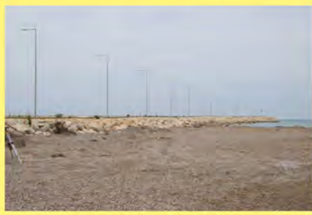
The area of the recently constructed harbour of Lechena (2005). The eastbound coastline has changed dramatically by the deposition of coastal sediments and algae. This progradation at this part reached the 50 meters and was mapped very accurately with the RTK-GPS methodology.
