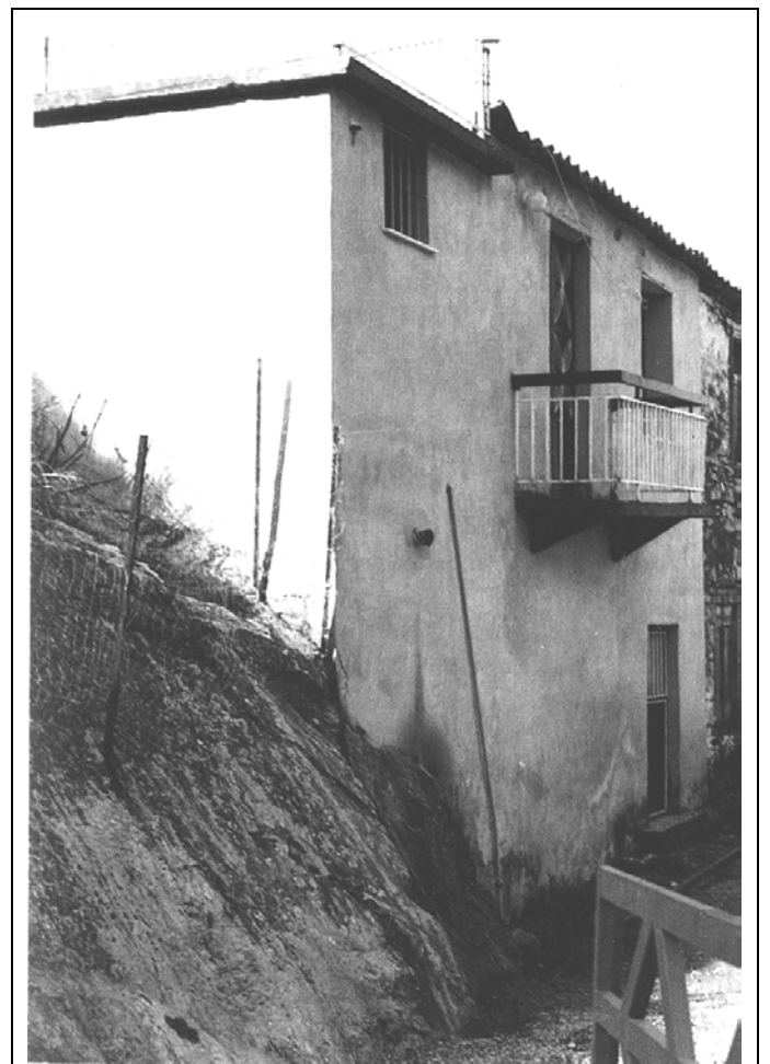
Figure 4 Two old houses remained untouched after the earthquake, although they have been built on an old inactive fault surface but on a massive rock body (neritic carbonates)
