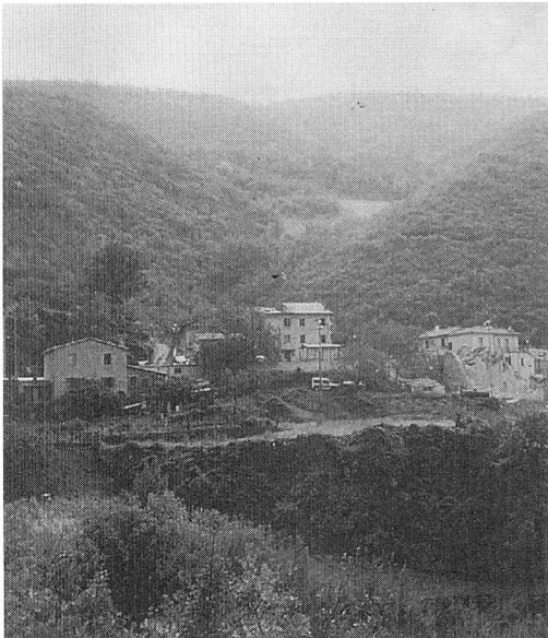
Figure 6. View of a built-up unit in the broad region of Nocera Umbria-Baghara, which suffered significant damages and was based on talus scree.
